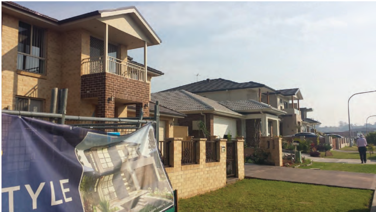
Figure 11.1: Newly constructed houses in Flynn Avenue, currently acting as a major thoroughfare. There is no formed footpath and no footpath area on the other side of the road. There is no footpath on either side of the road in undeveloped areas to the east.
