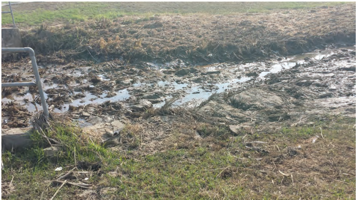
Figure 11.5: The drainage reserve showing recent maintenance activities.
