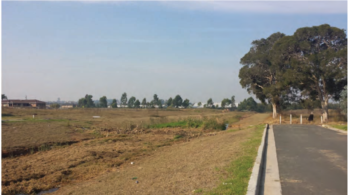
Figure 11.6: The drainage reserve showing recent maintenance activities. Erosion of the channel is evident, as are areas of bare earth and rubbish in the drain. Middleton Grange Primary School is in the distance. The narrow road should be noted including the absence of a footpath and pedestrian access to the school.
